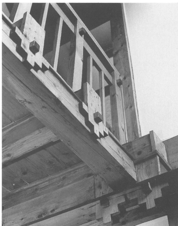
6 Charles-Edouard Jeanneret, Villa Fallet, La Chaux-de-Fonds, 1906–7. Detail of staircase-landing
